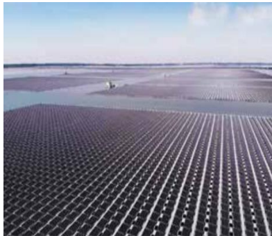
13.5 MW Floating PV (Japan)
